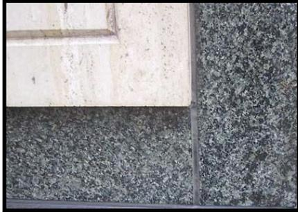
building stone, a rock known in the construction trade as Verde Fontaine. South African quarries produced this pine green rock, which solidified underground over one billion years ago. The green coloration comes from the mineral chlorite, which forms from the alteration of iron- and magnesium-rich minerals within the rock. (The tan rock is Italian travertine.)
