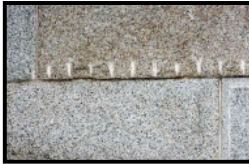
An example of the Tarbox cutting method.
